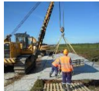
HEAVY-DUTY MACHINERY PARKING SITES
