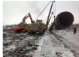
TEMPORARY ROADS FOR HEAVY MACHINERY
