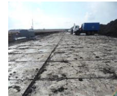
HEAVY MACHINERY AND VEHICLE PARKING SITES
